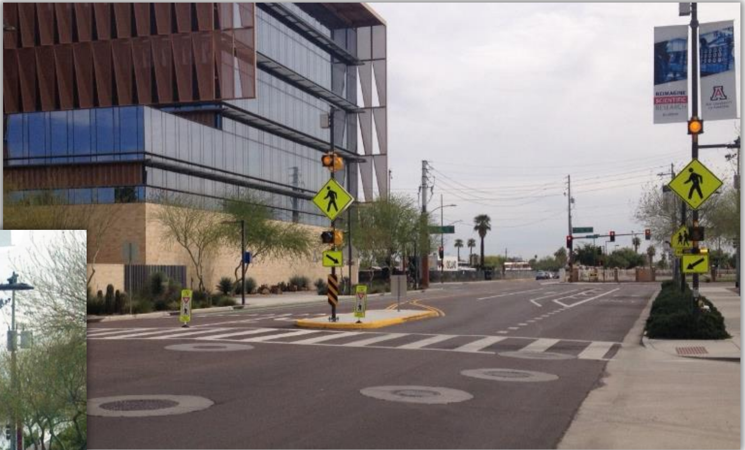
Pedestrian Flashing Beacon (PFB) North Fillmore Street and 6 th Street
