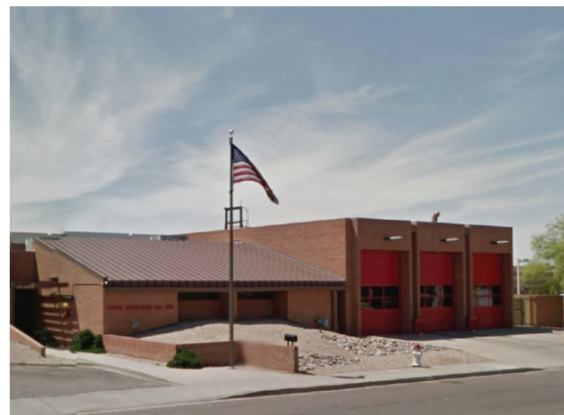
Phoenix Fire Department, Station 23
