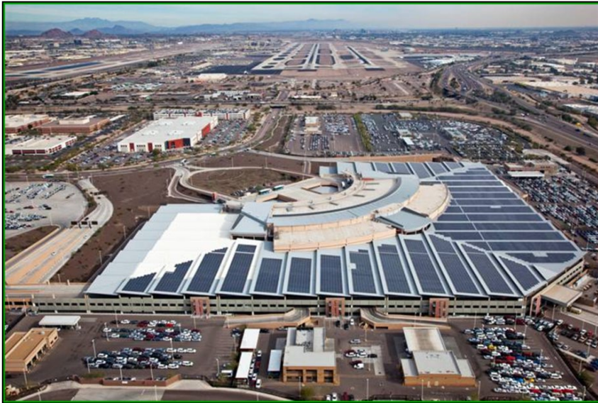
Rental Car Center Solar Installation: 4.2 MW
