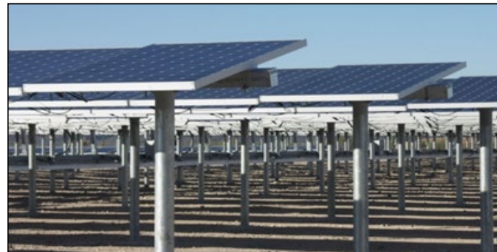
Lake Pleasant Water Treatment Plant – 7.5 MW
