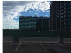
06: EXISTING SITE PHOTO
