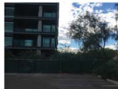
05: EXISTING SITE PHOTO
