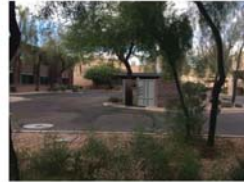
08: EXISTING SITE PHOTO
