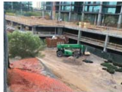
11: EXISTING SITE PHOTO
