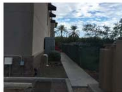
09: EXISTING SITE PHOTO
