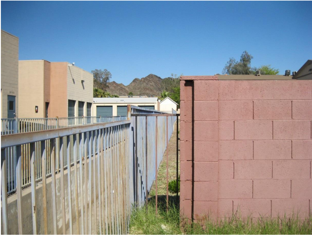
6: Northeast corner of property looking east
