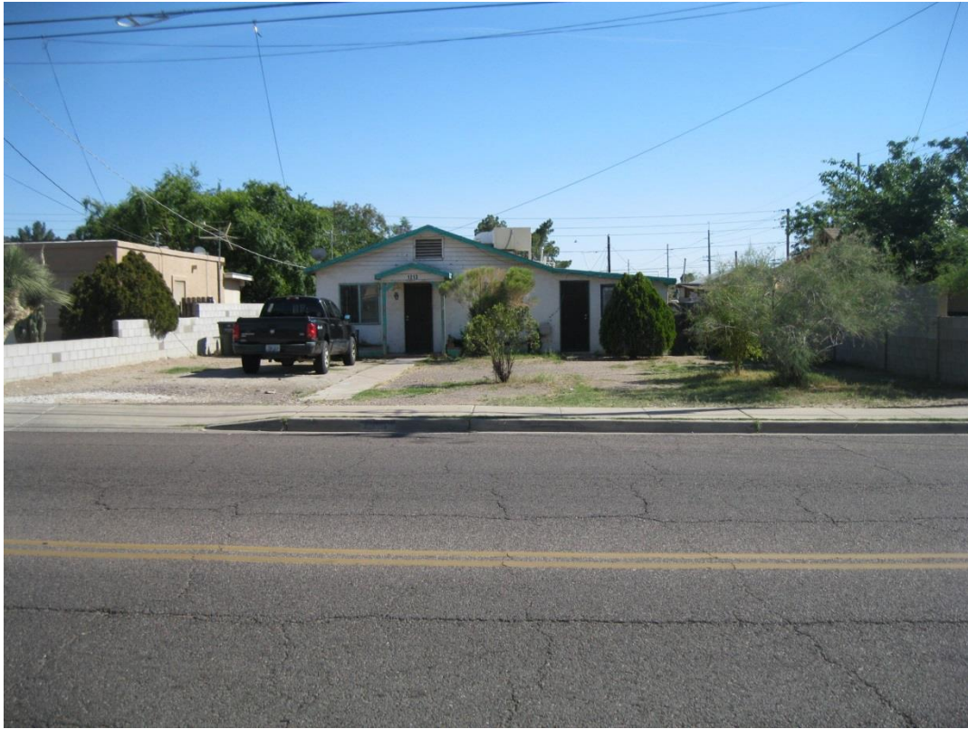
11: Southeast corner of property looking south
