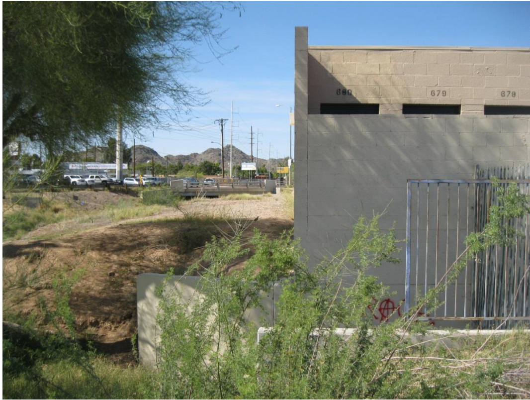
1: Northwest corner of property looking north
