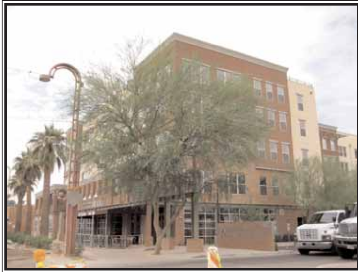
The Cheuvront Wine and Cheese Café and Artisan Lofts development illustrates the buildings closer to the street
