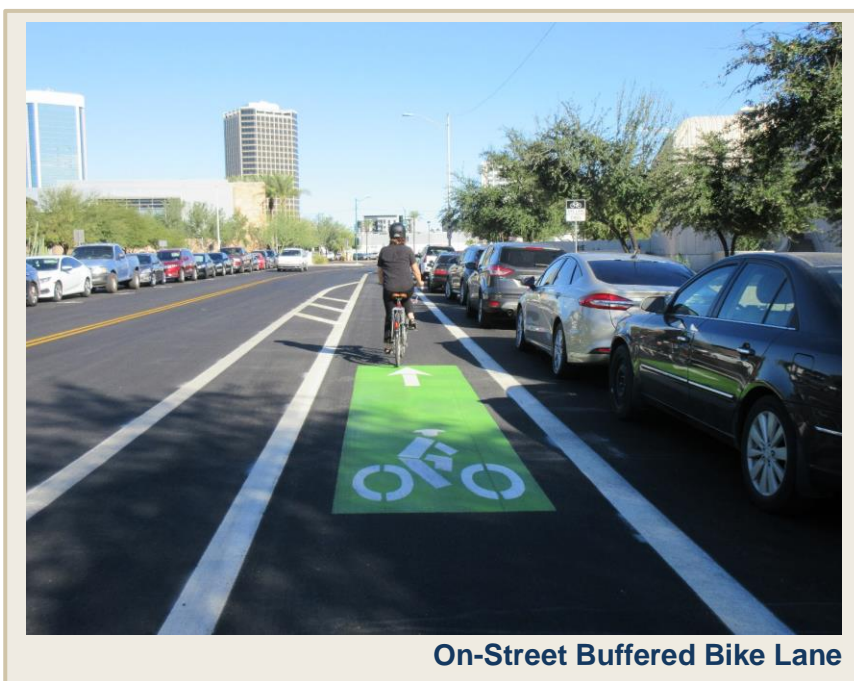
Figure 8.5-2 On-Street Buffered Bike Lane
