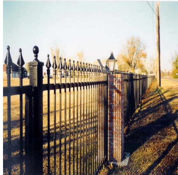
Wrought-iron fencing (Figure 4)
