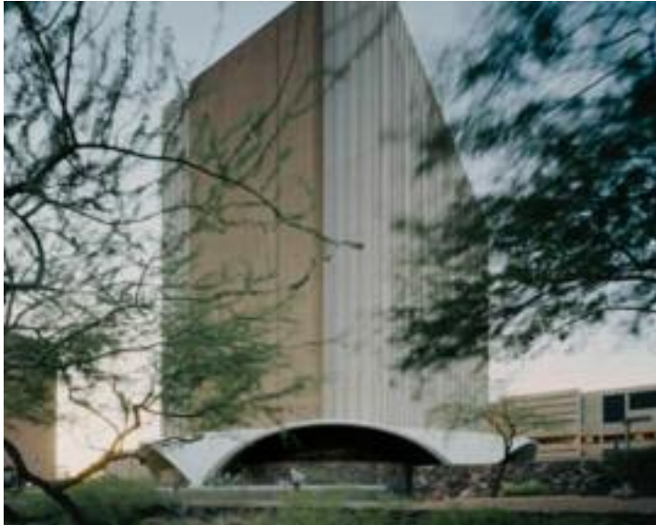
County Supervisors Auditorium and Office, (1962, 1973) 205 West Jefferson Street
