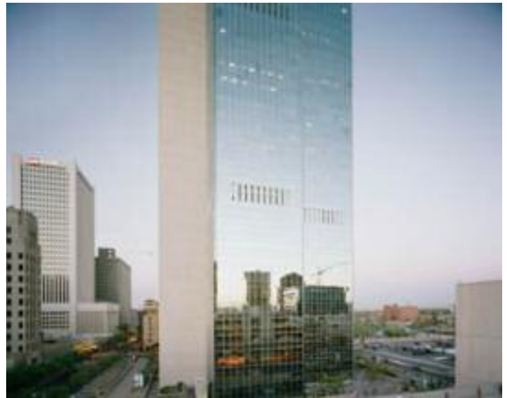
Valley Center/Chase Tower, (1972) 201 North Central Avenue
