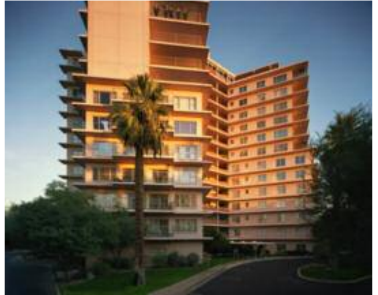
Phoenix Towers, (1956) 2201 North Central Avenue
