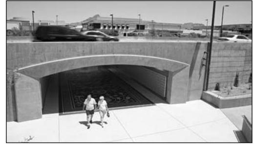
The Street Transportation Department opened the Camelback Pedestrian Underpass, which connects the north and south shopping areas at Camelback Road, east of 24th Street.
