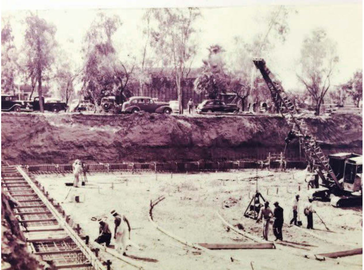
1947 Construction of Clarifier at 23rd Avenue WWTP
