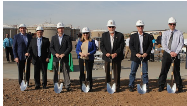
The Biogas project is expected to produce $1.2 million in annual revenue, to be shared among the cities that jointly own the 91st Avenue Wastewater Treatment Plant.
