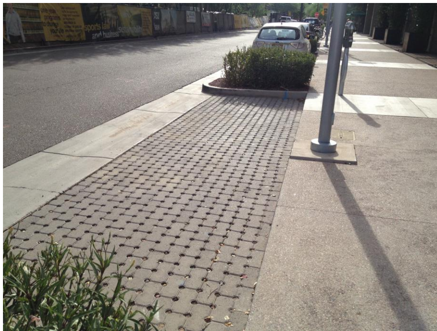
Figure 7: Pervious Pavers (Interlocking Porous Concrete Pavers) Source: City of Phoenix, Office of Environmental Programs.
