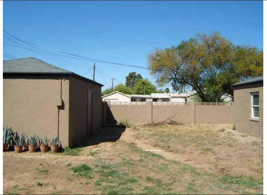
View facing west: garage addition to be constructed on north side of existing garage
