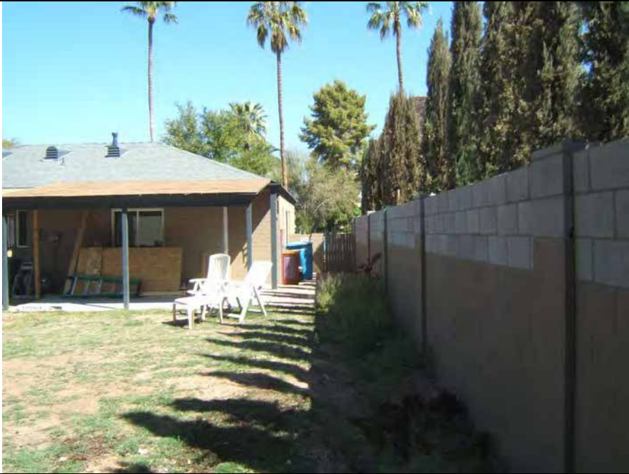
View facing north: location of proposed 8' wide concrete slab in back yard
