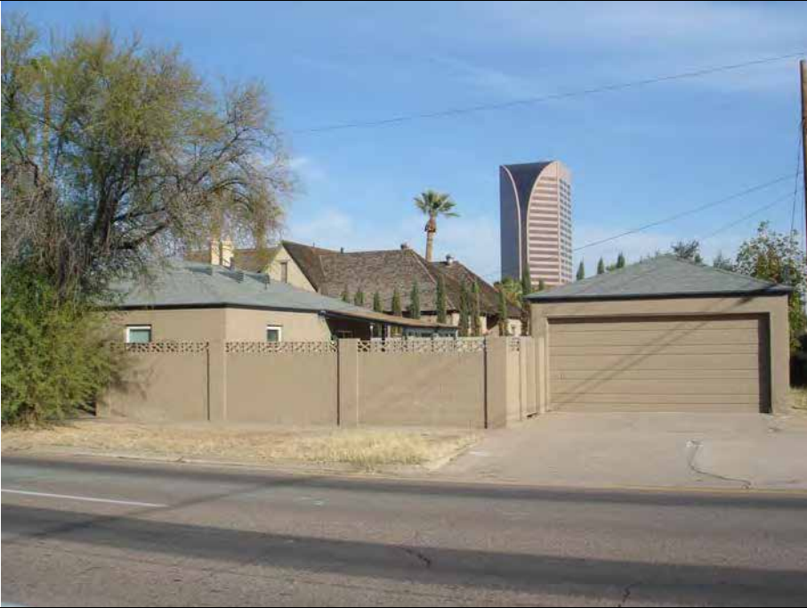
View facing N/NE: detached rear garage and house
