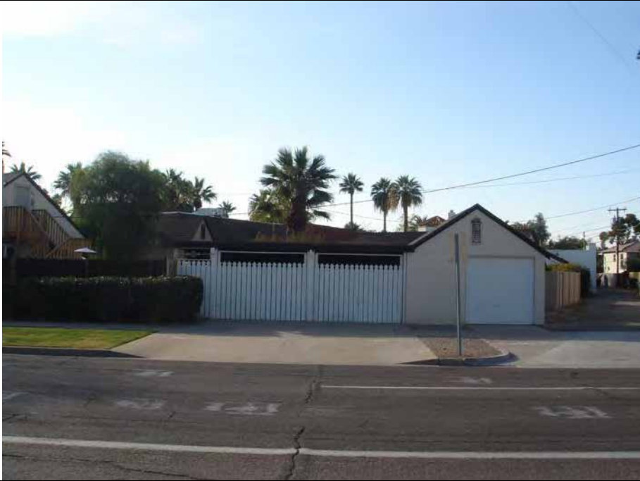
Corner house with carport addition and new side driveway at 3 rd Ave. & Monte Vista Rd.
