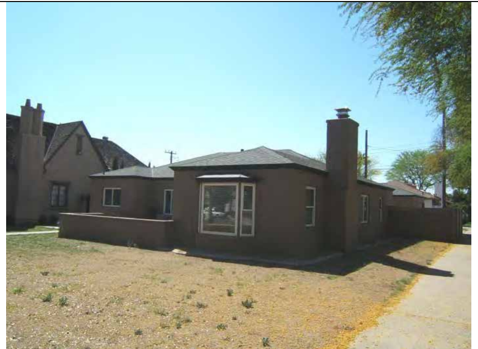
View facing S/SE: house with detached garage at rear
