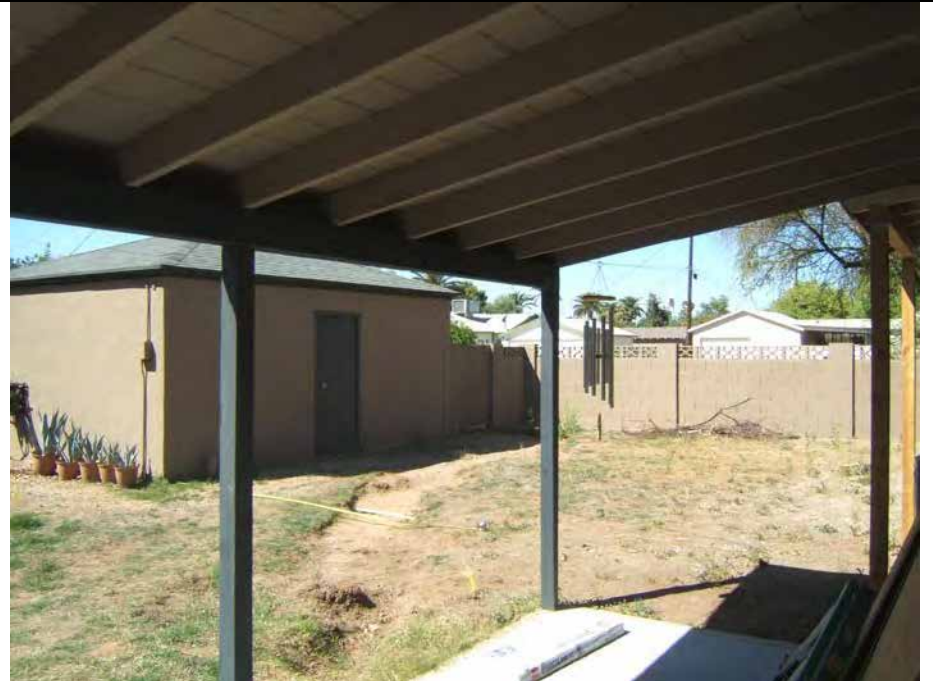
View facing S/SW: general area where garage addition to be built
