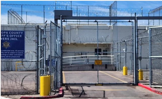
TOWERS SECURE GATE
