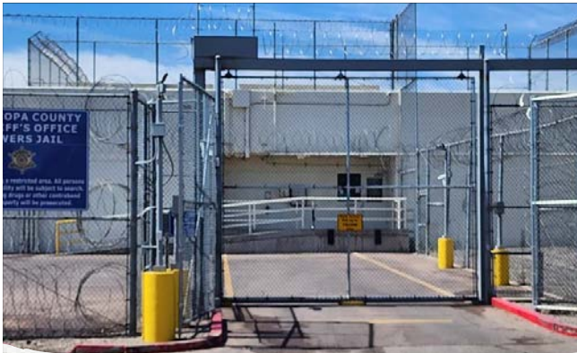
TOWERS SECURE GATE
