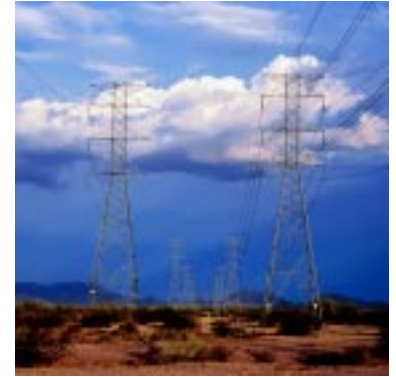
Figure 3.26 Existing utility corridors provide opportunities for regional trail connections
