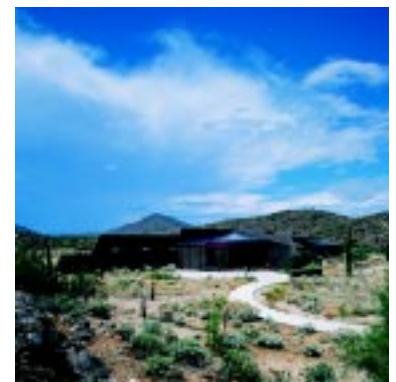
Figure 3.27 South Mountain Park's new environmental education center
