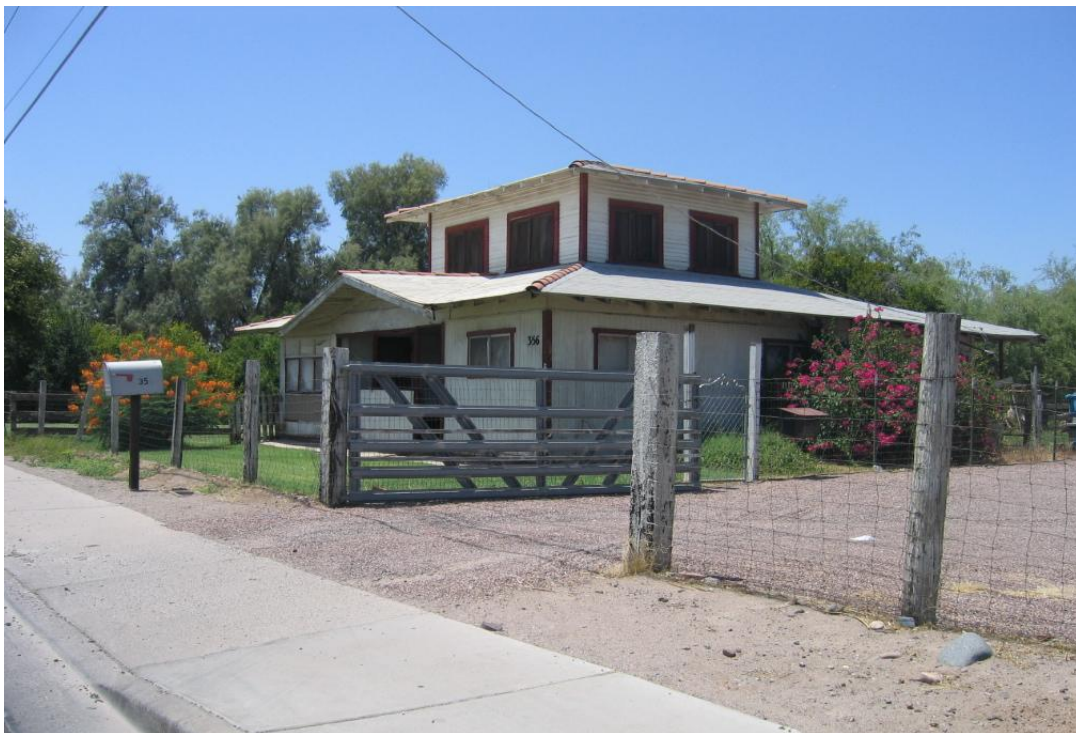
Figure 16. Vernacular Farm Cottage at 356 W. Broadway Road.
