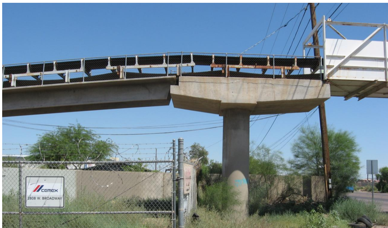
Figure 25. Elevated gravel conveyor over Broadway Road west of 27 th Avenue.
