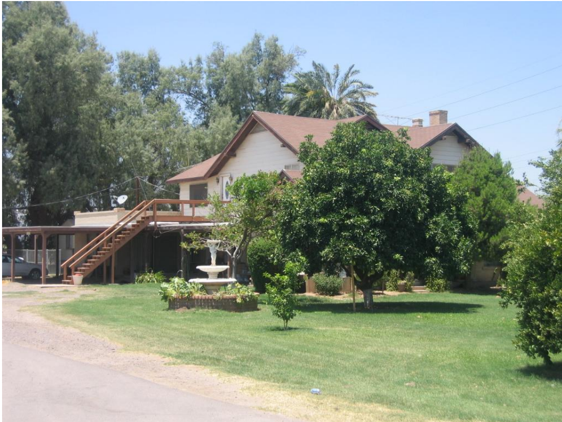
Figure 17. Bungalow Farmhouse at 4812 S. 43 rd Avenue.
