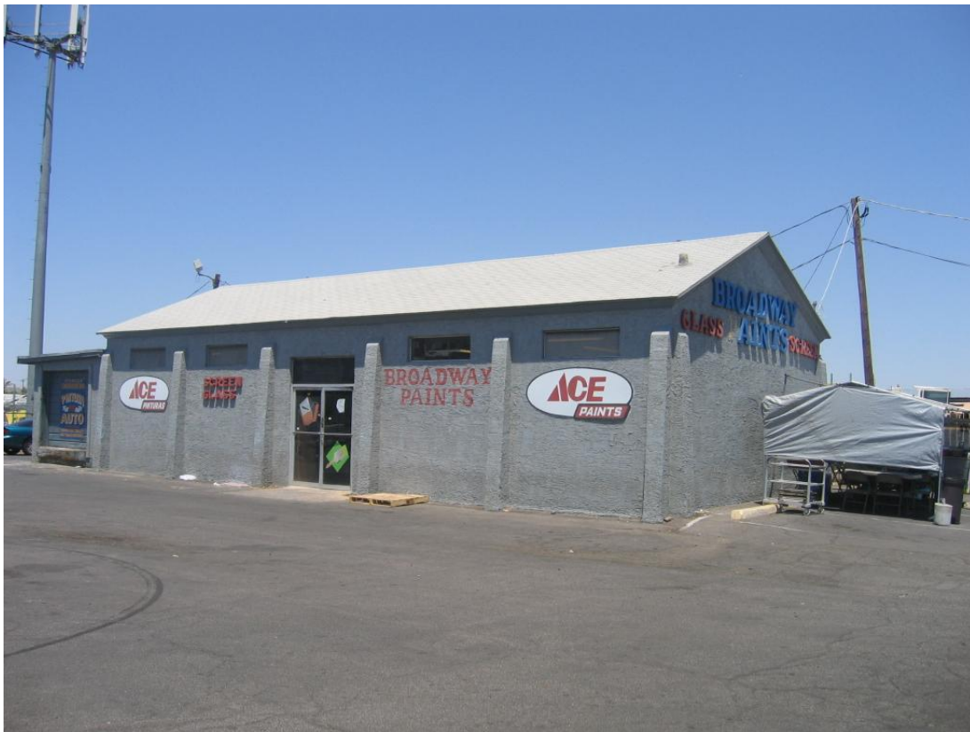
Figure 36. Former Broadway Methodist Church building at 32 E. Broadway Road.
