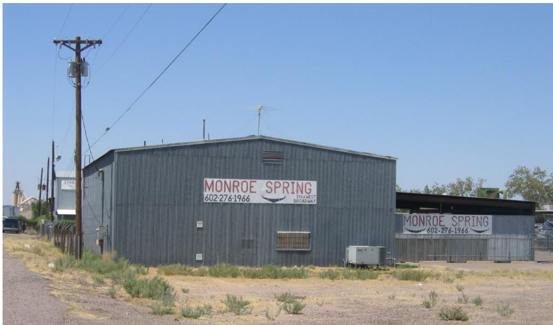
Figure 22. Monroe Spring building at 1966 W. Broadway Road.
