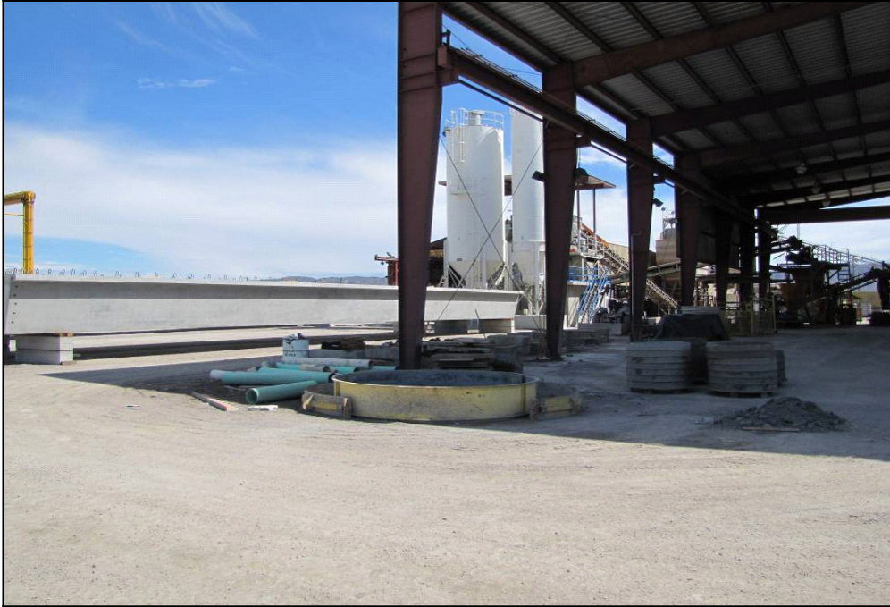
Smith Septic Tank/Smith Pre-Cast Co., batch plant.
