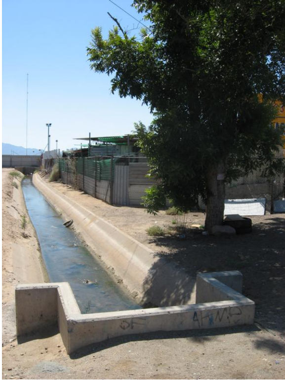
Figure 12. Open irrigation ditch east of 2935 W. Broadway Road (left).
