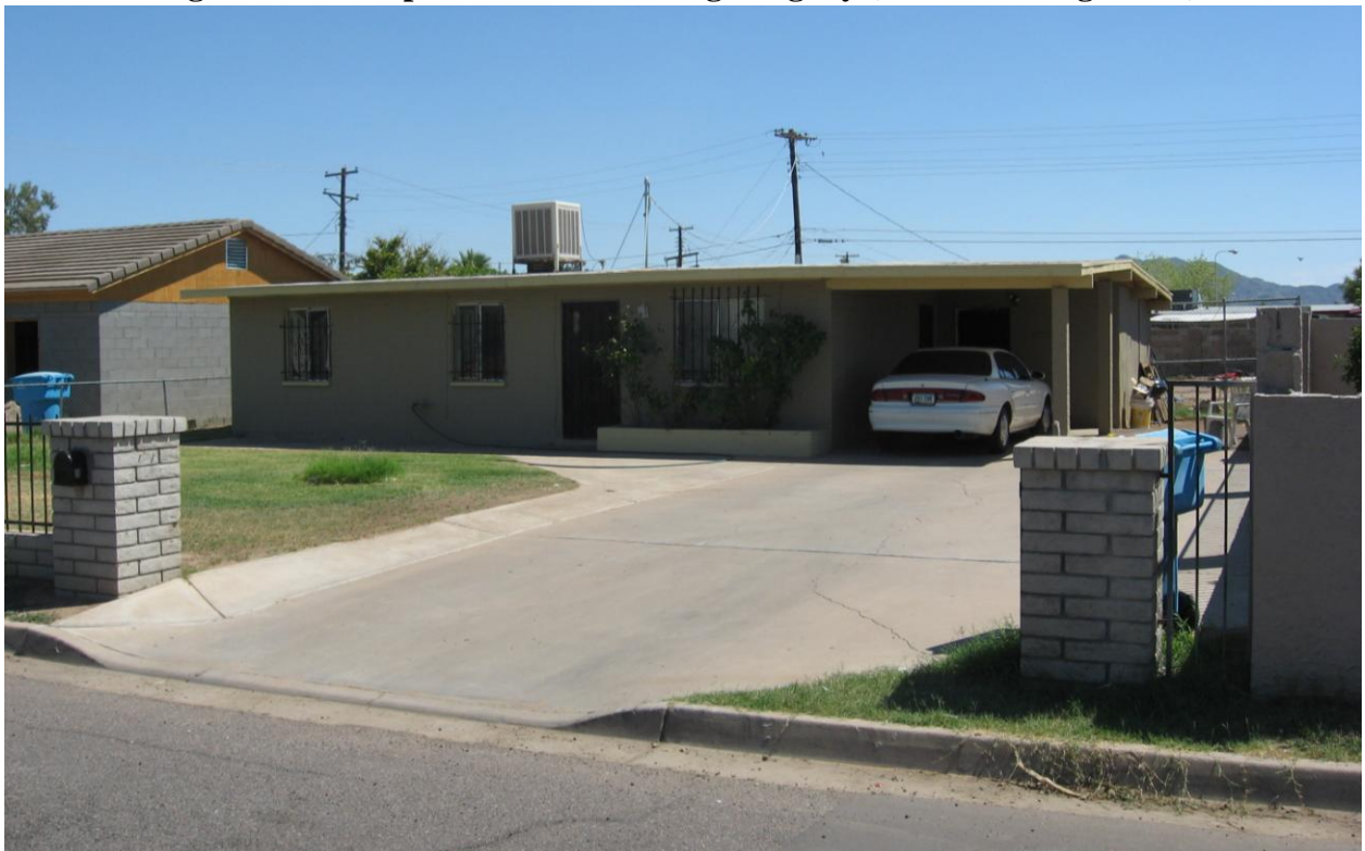
Figure 32. Example of a house retaining integrity (Lot 188 on Figure 32).
