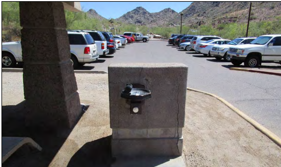
Figure 3. Photograph of the concrete water fountain, parking lot, and street lights of Building Group 1. View facing east.
