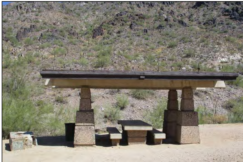
Figure 6. Photograph of Building 2A, a ramada of Building Group 2, view facing north.
