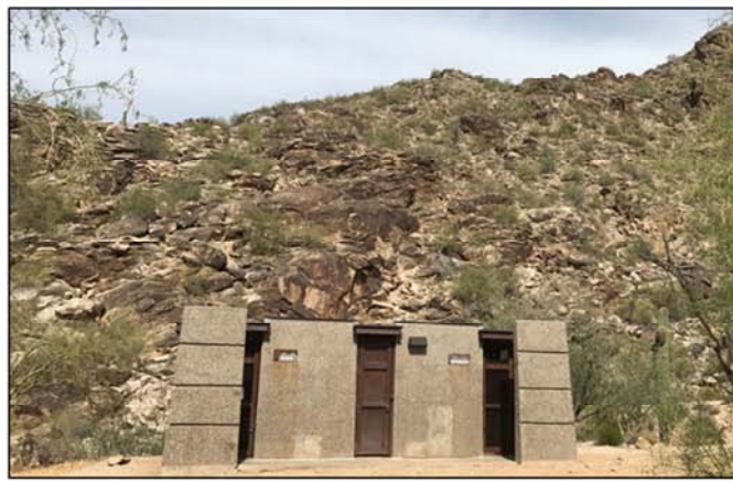
Photograph of a restroom facility near the Piedras Grandes recreation area at South Mountain Park. View facing east.
