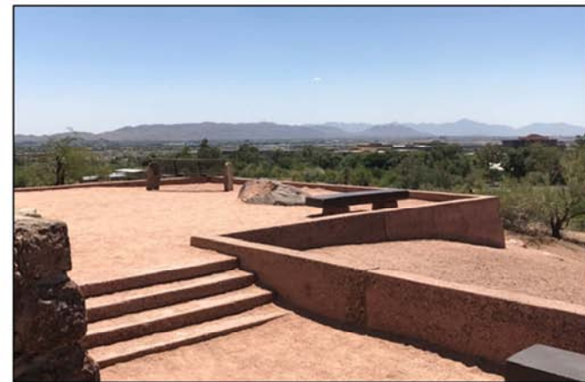
Photograph of the exposed aggregate retaining walls at Hunt's Tomb, view facing southwest.
