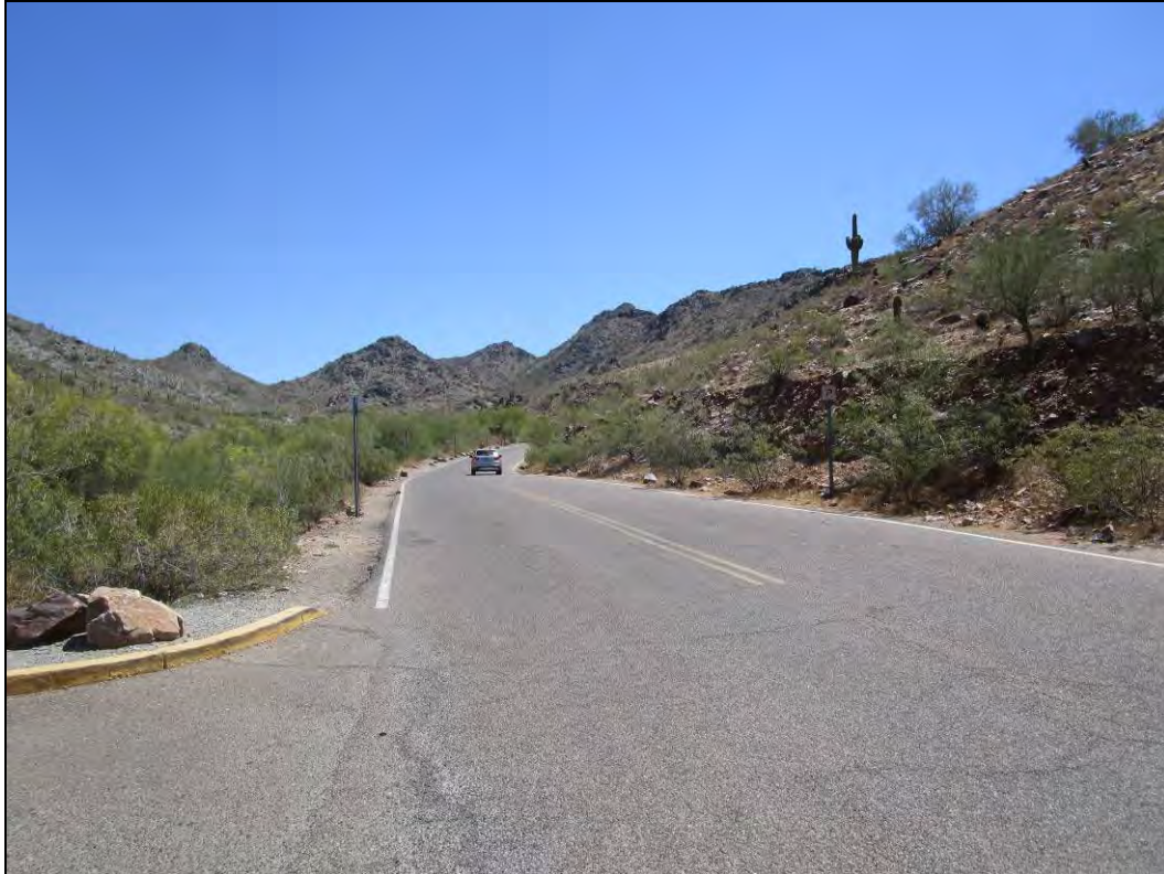
Figure 5. Overview of the main access road from the west end of the recreation area, view facing northeast.
