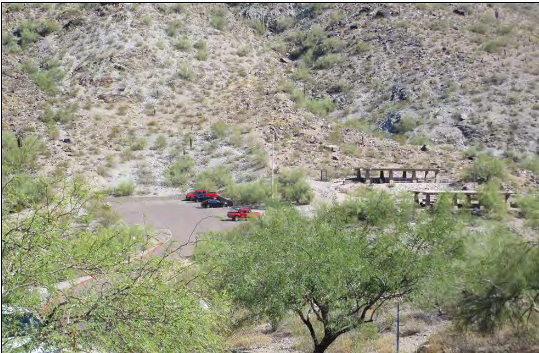
Figure 1. Overview of Building Group 5, from the slopes of Building Group 4, view facing northeast.
