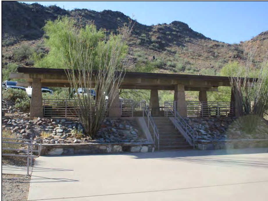
Figure 1. Overview of Building 6B, a 60-capacity ramada of Building Group 6, view facing south.
