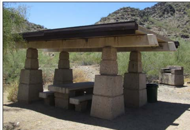
Photograph of the a small ramada and barbeque at Area 9 of North Mountain Park, view facing southwest.
