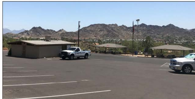
Photograph of modern facilities at North Mountain Park, including a Ranger Station and two ramadas, view facing southeast.
