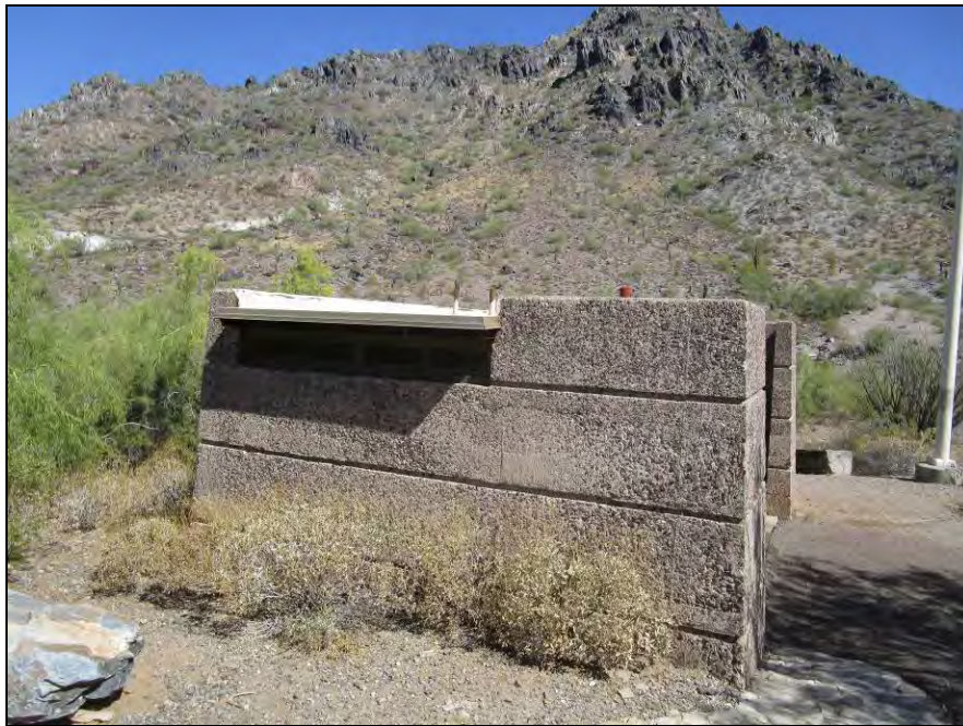
Figure 1. Photograph of the north façade of Building 8, showing the slightly protruding roof over the open window. View facing north.
