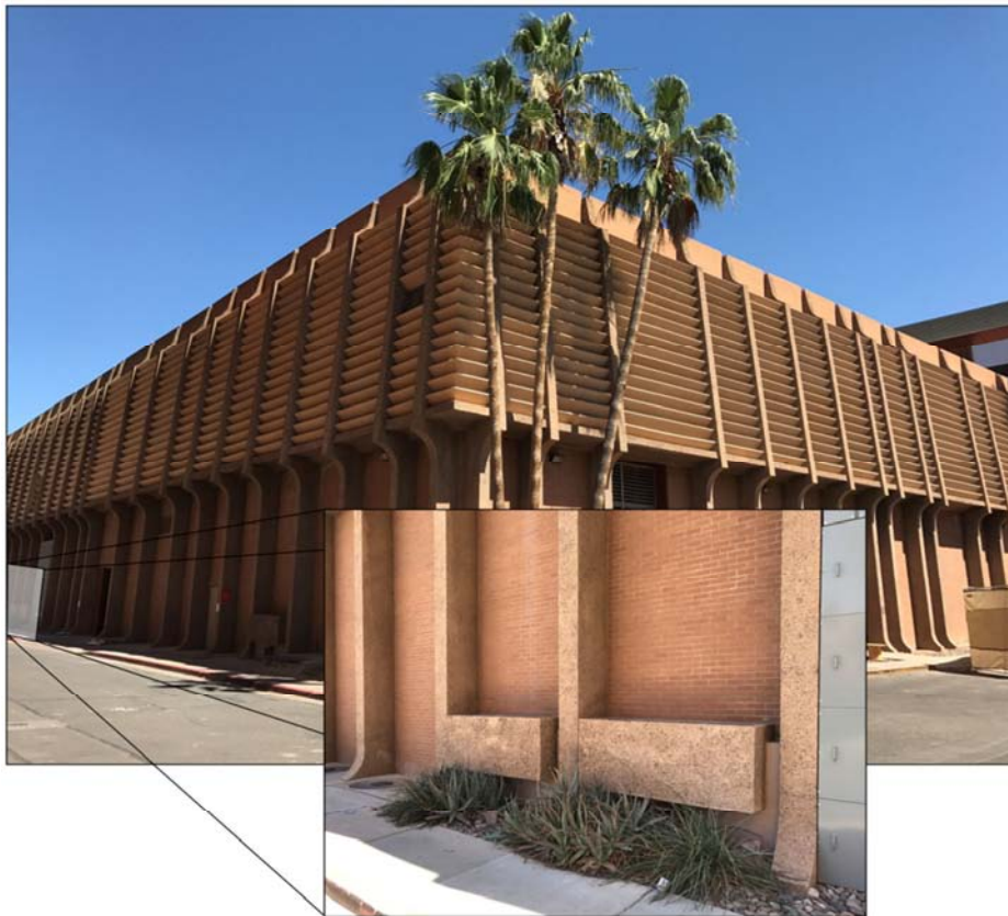
Figure 13. Photograph of the Central Plant at Arizona State University, constructed in 1968.
