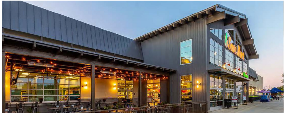
Distinctive entryways, metal accents, building offsets and articulation
