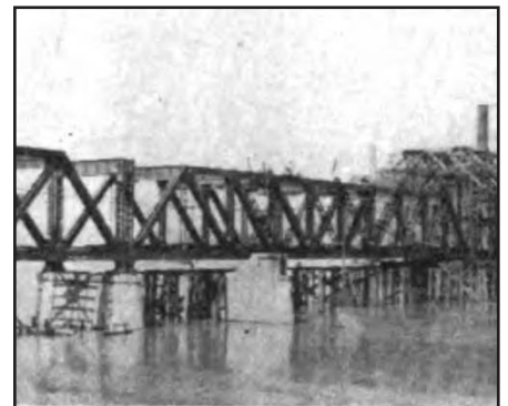
Central Avenue Bridge
