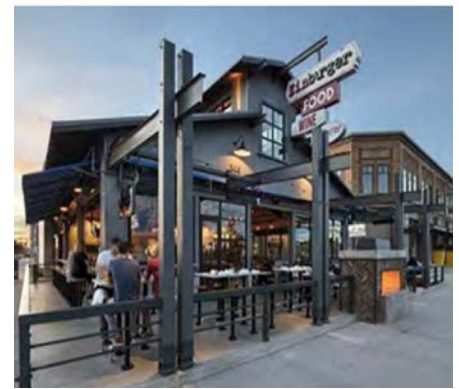
Distinctive rooflines, rafter beams
