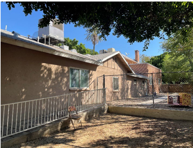
Side (south) façade of main house, including rear additions, view northeast.
