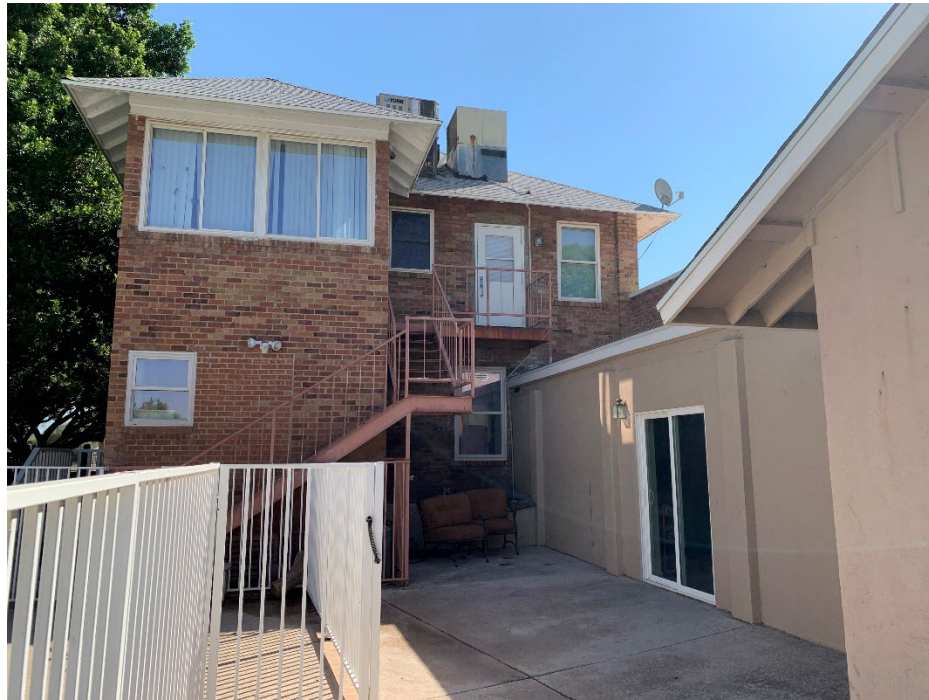
Rear (west) façade of main house, including rear additions, view east.
