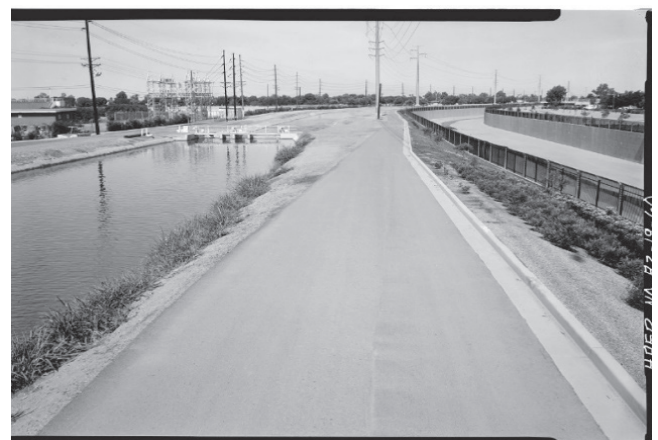
Low level check station on the Arizona canal, near the Deer Valley Water Treatment Plant. Library of Congress Historic American Engineering Record, 1990.
