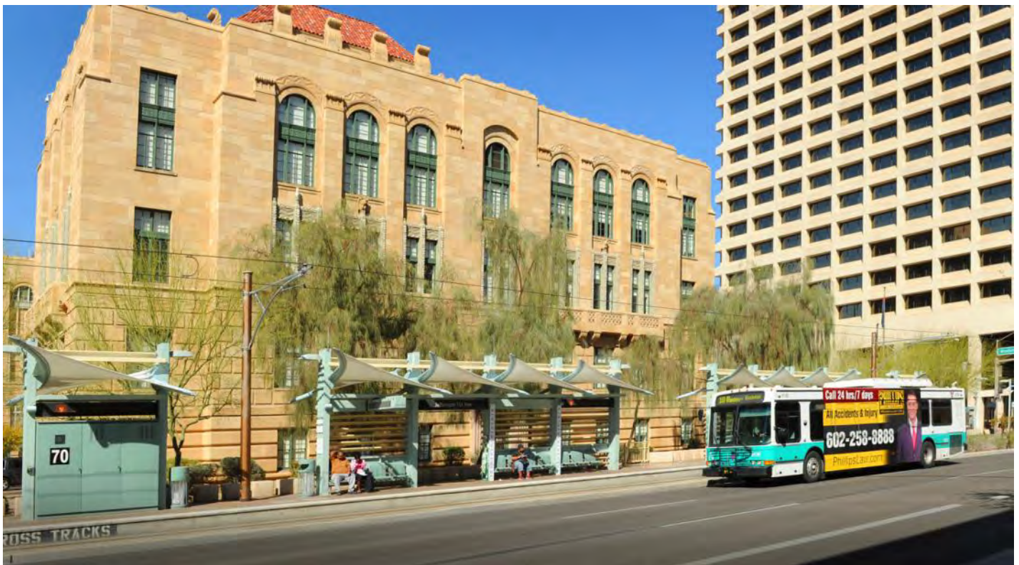
The Route 10 serves the current City of Phoenix Courthouse on Jefferson Street.
