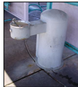
Figure 3.10 The drinking fountain at the Desert Sky Mall Transit Center lacks the ADA-required dual-height fountains.
