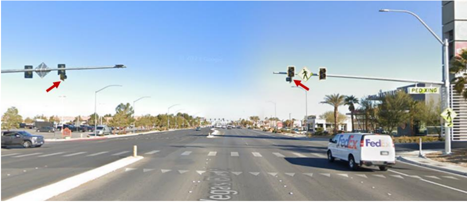
(a) Vehicle View of Installation
