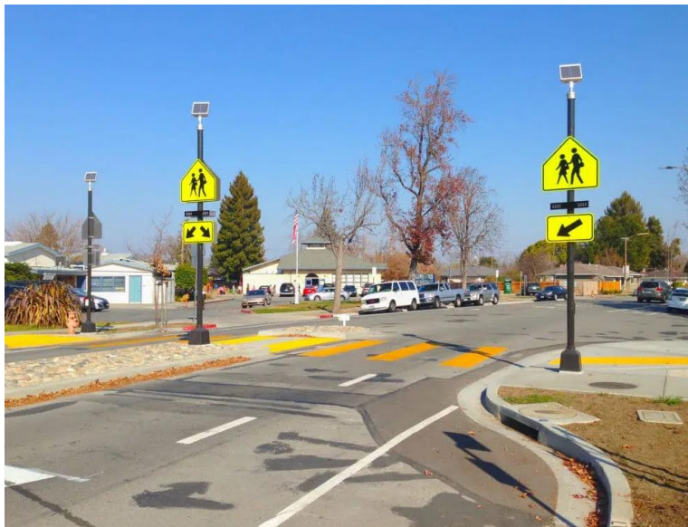
Figure 10: Rectangular Rapid Flashing Beacon
